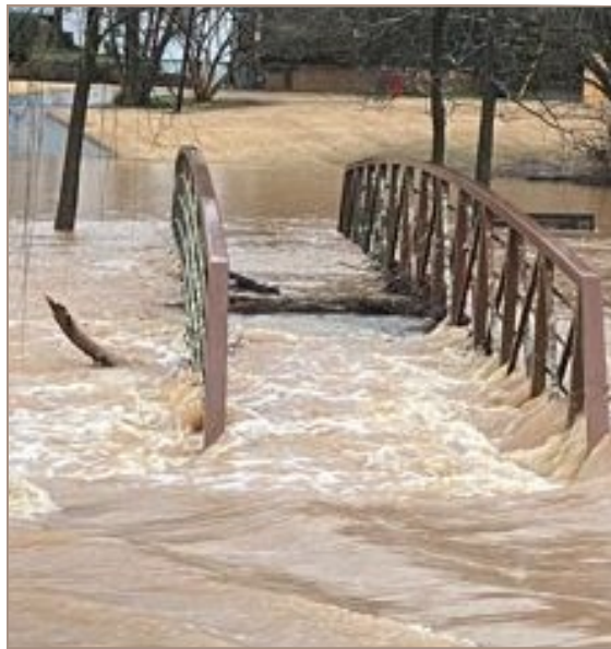
The photo to the left from Mike Womack shows the footbridge next to Veteran's Park.
